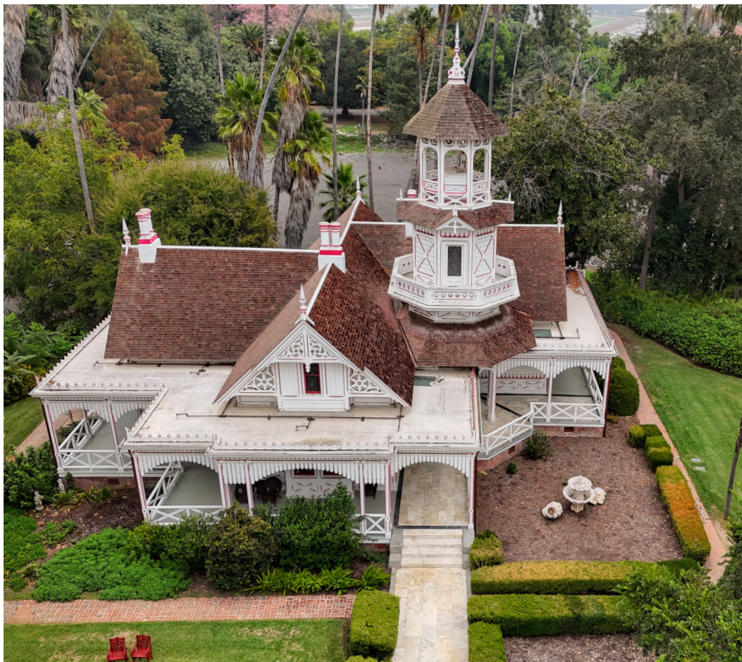
An aerial view of the Cottage after the restoration. The tower and cupola (top) needed stabilization and the steps serious repairs.
